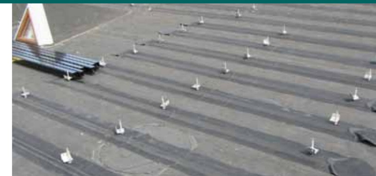
Wooden bars inserted on the roof with hangerbolts for mounting frame support
