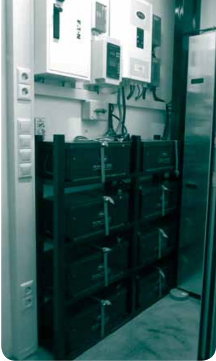
Typical example of an AGM battery bank, powering a 3.5 kW inverter
